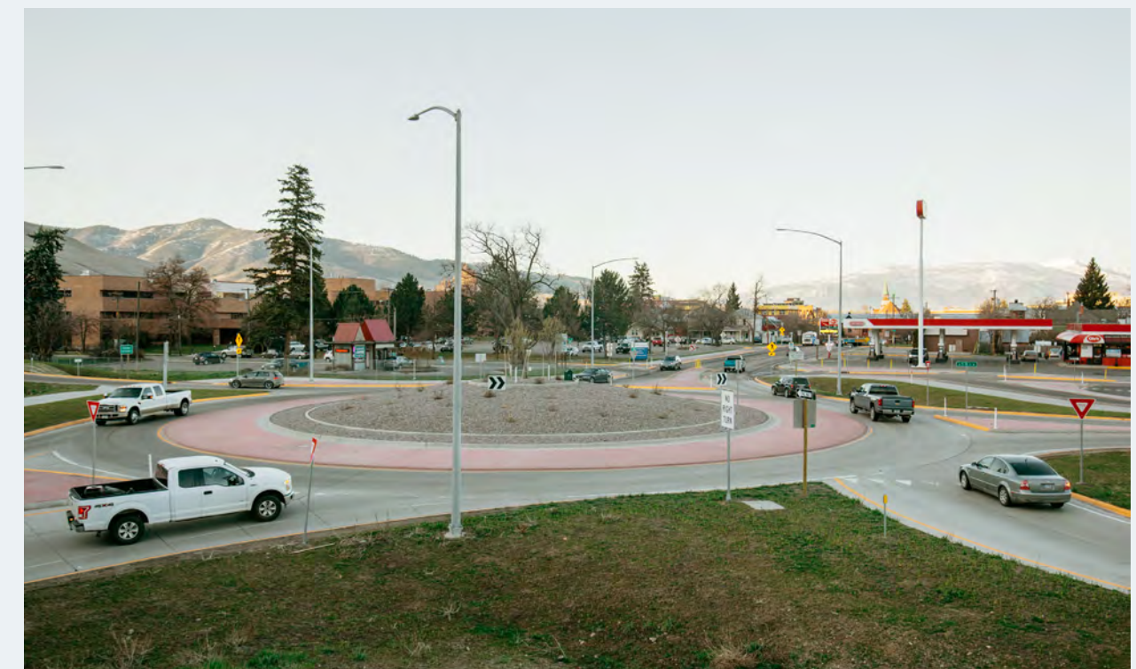
MDT constructed safety improvements at the Orange Street interchange of I-90
