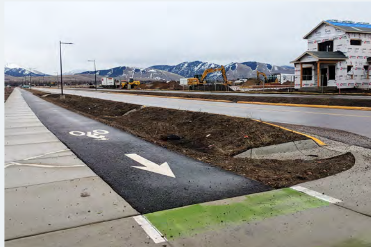
Preliminary S w tpqyen area complete streets construction
