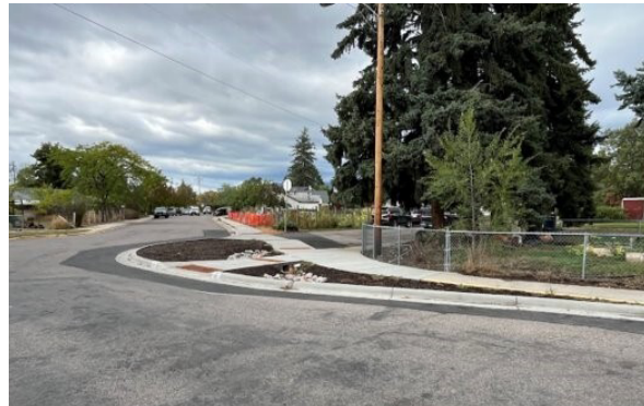
Curb extensions built as part of the Ivy Street/Franklin Neighborhood Greenway
