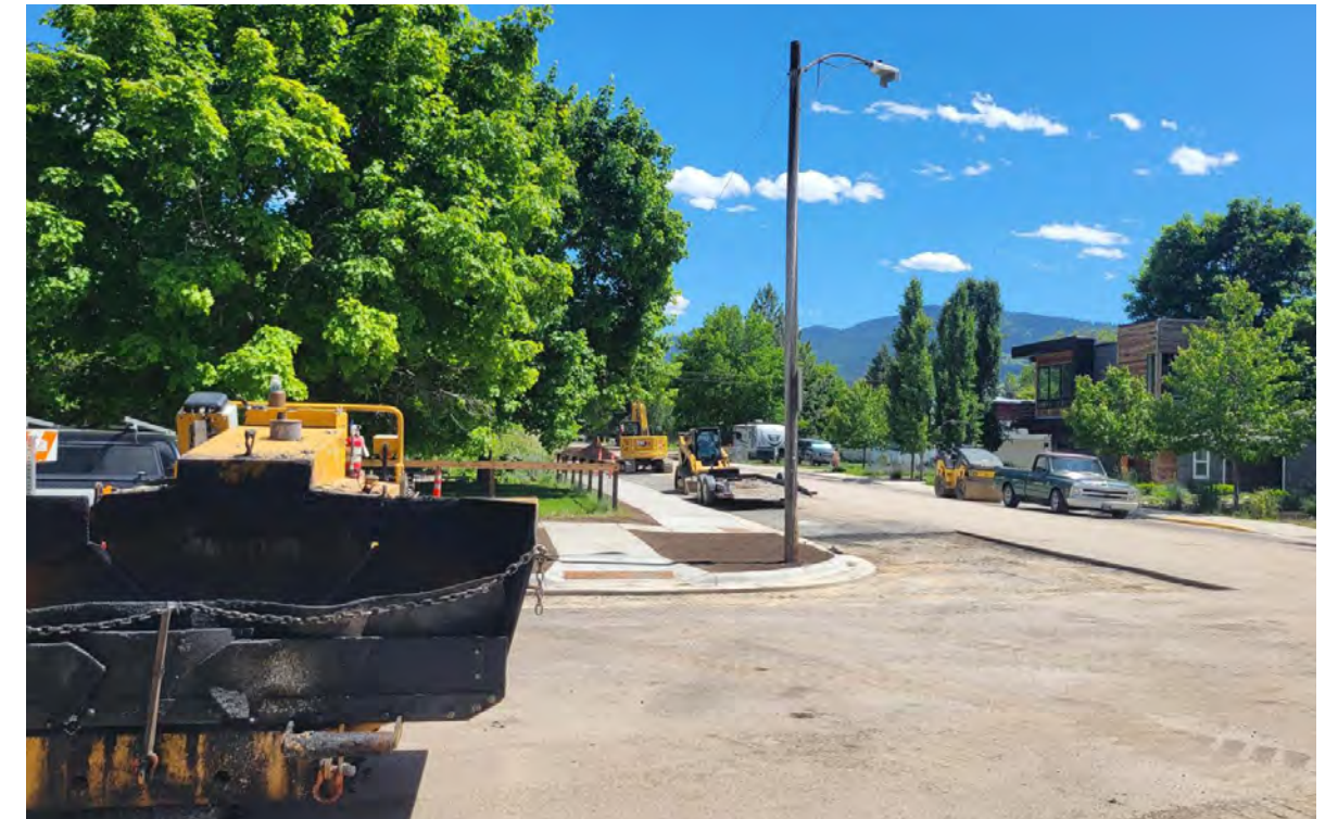
Construction of the Ivy Street/Franklin Neighborhood Greenway
