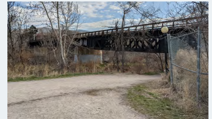
Existing Montana Rail Link Trestle
