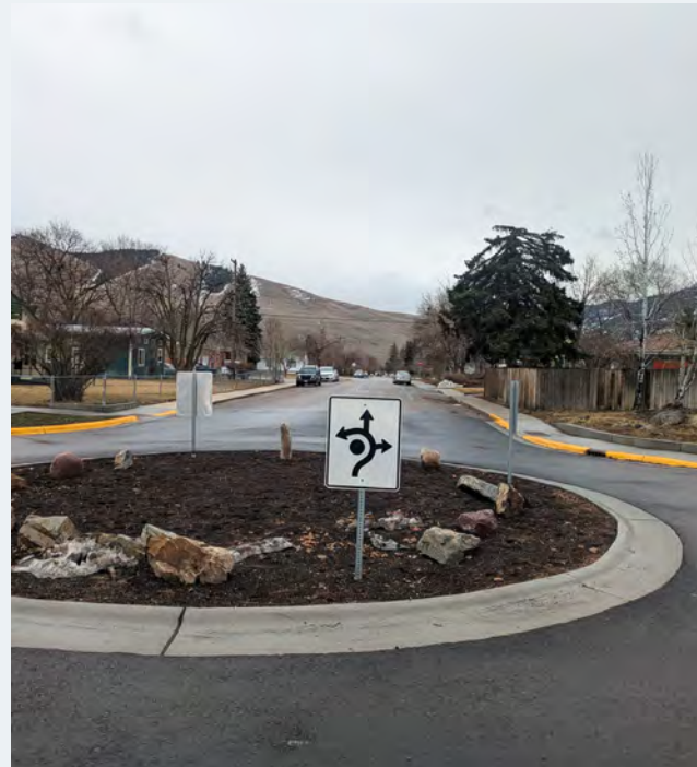
Installed neighborhood greenway elements
