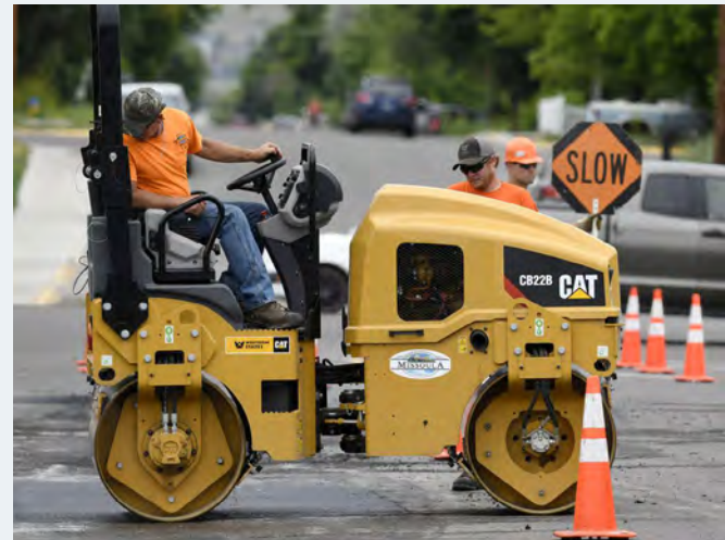
Construction work in Missoula
