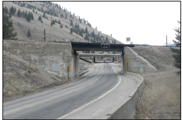
Photo 3.1: Railroad Underpass Looking North
