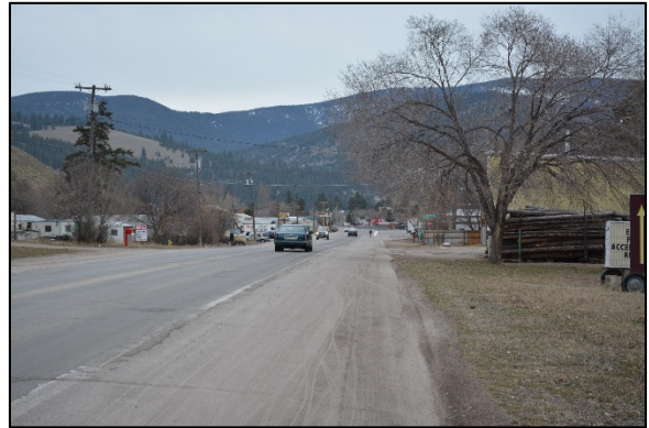
Photo 3.3: MT 200 Looking Northwest
