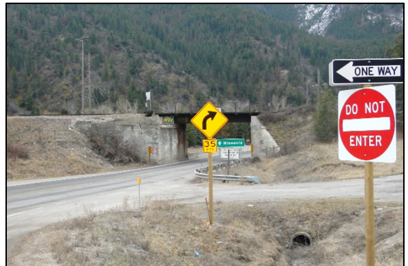
Photo 3.2: Looking South from Eastbound Off-ramp
