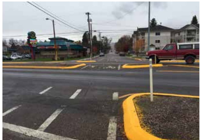
This bicycle crossing treatment along Burton Street across West Broadway Street represents what some of the seventy comments about new crossing treatments may be seeking.
