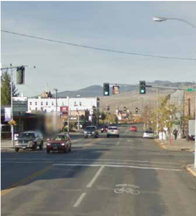
Bike routes are currently designated on many arterial and Collector streets where bike lanes are not feasible.
