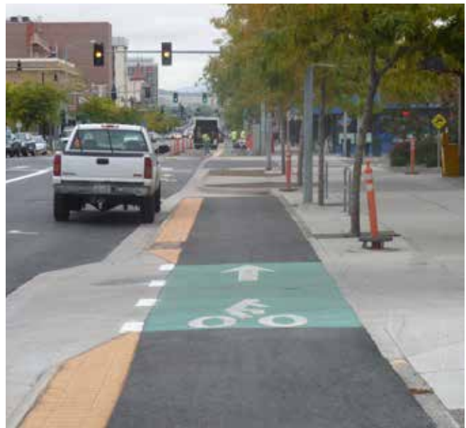
Raised one-way cycle track on Higgins Avenue
