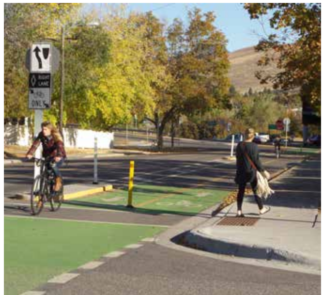
Street-level two-way cycle track on Maurice Avenue
