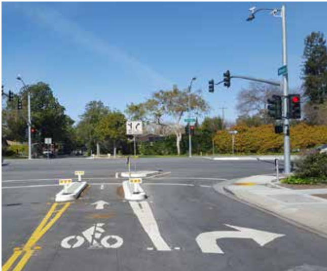
This spot treatment in Palo Alto, CA allows bicyclists to cross a major street without allowing through vehicle traffic on the local street network.
