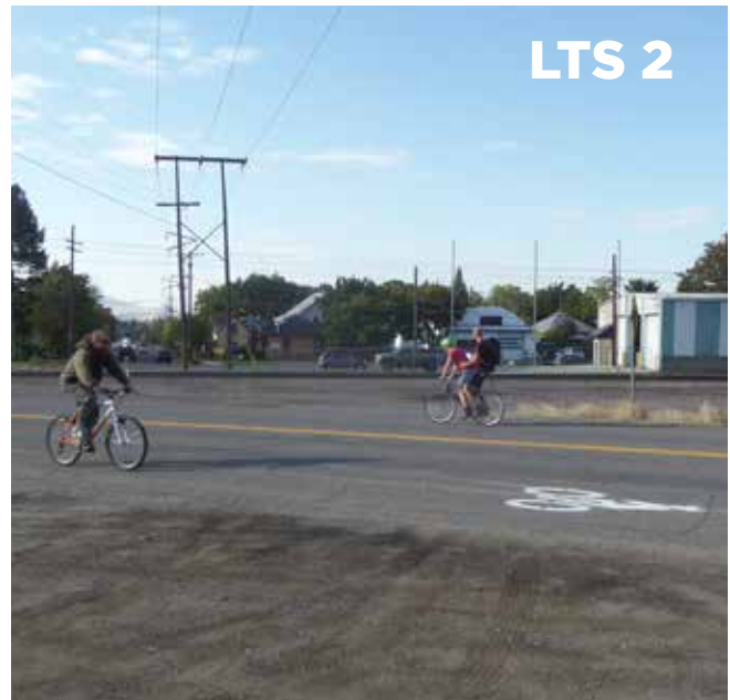
Bicycle lanes with no on-street parking and moderate speeds/volumes can be attractive for the mainstream population, as in this example on North 2nd Street near Greenough Drive).
