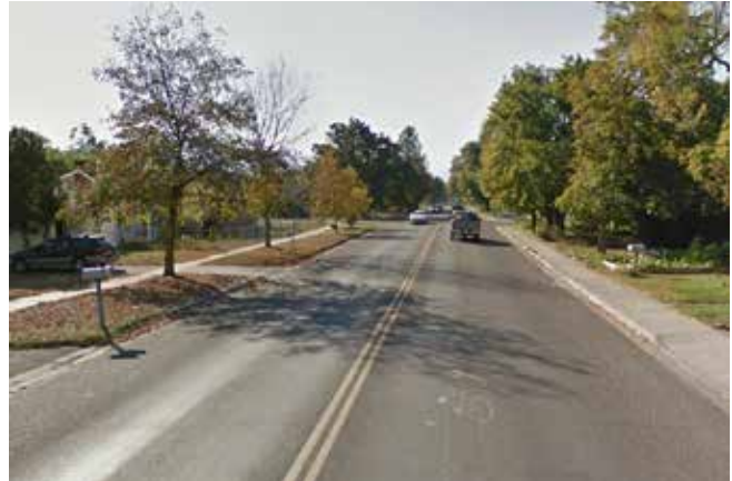
South 14th Street is designated as a bike route but carries heavy traffic and is uncomfortable for many bicyclists.
