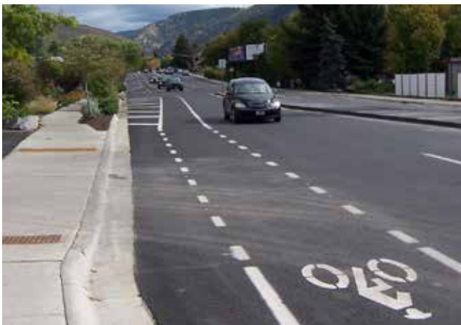
Bike lanes, if applied during routine pavement preservation projects or reconstructions carry very little cost
