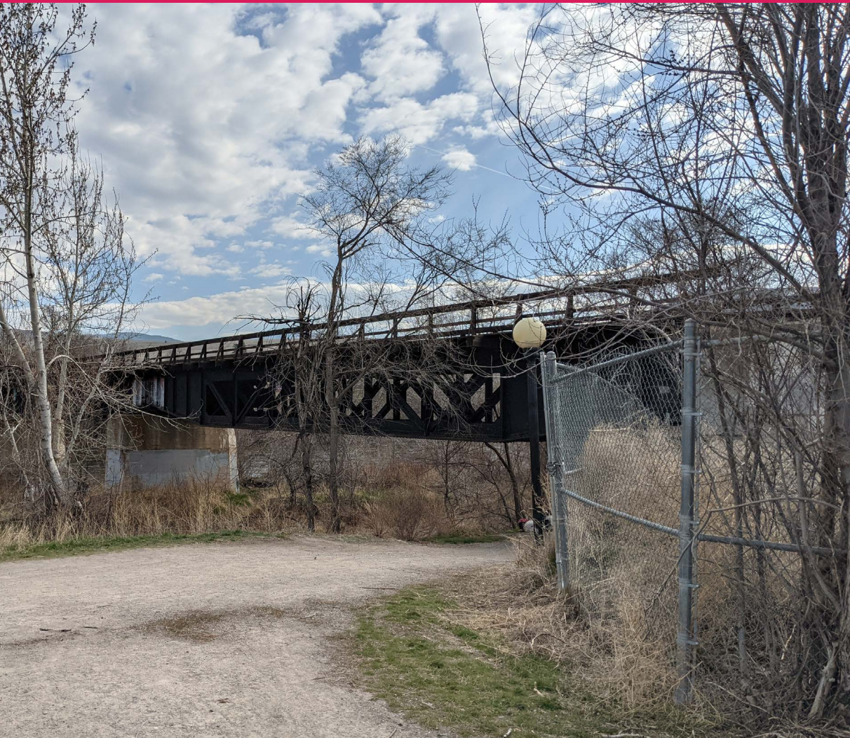
Existing Montana Rail Link Trestle
