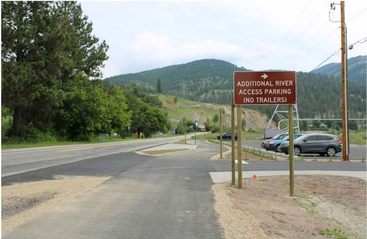
New parking area for Sha-Ron river access from Highway 200 between East Missoula and Bonner.
